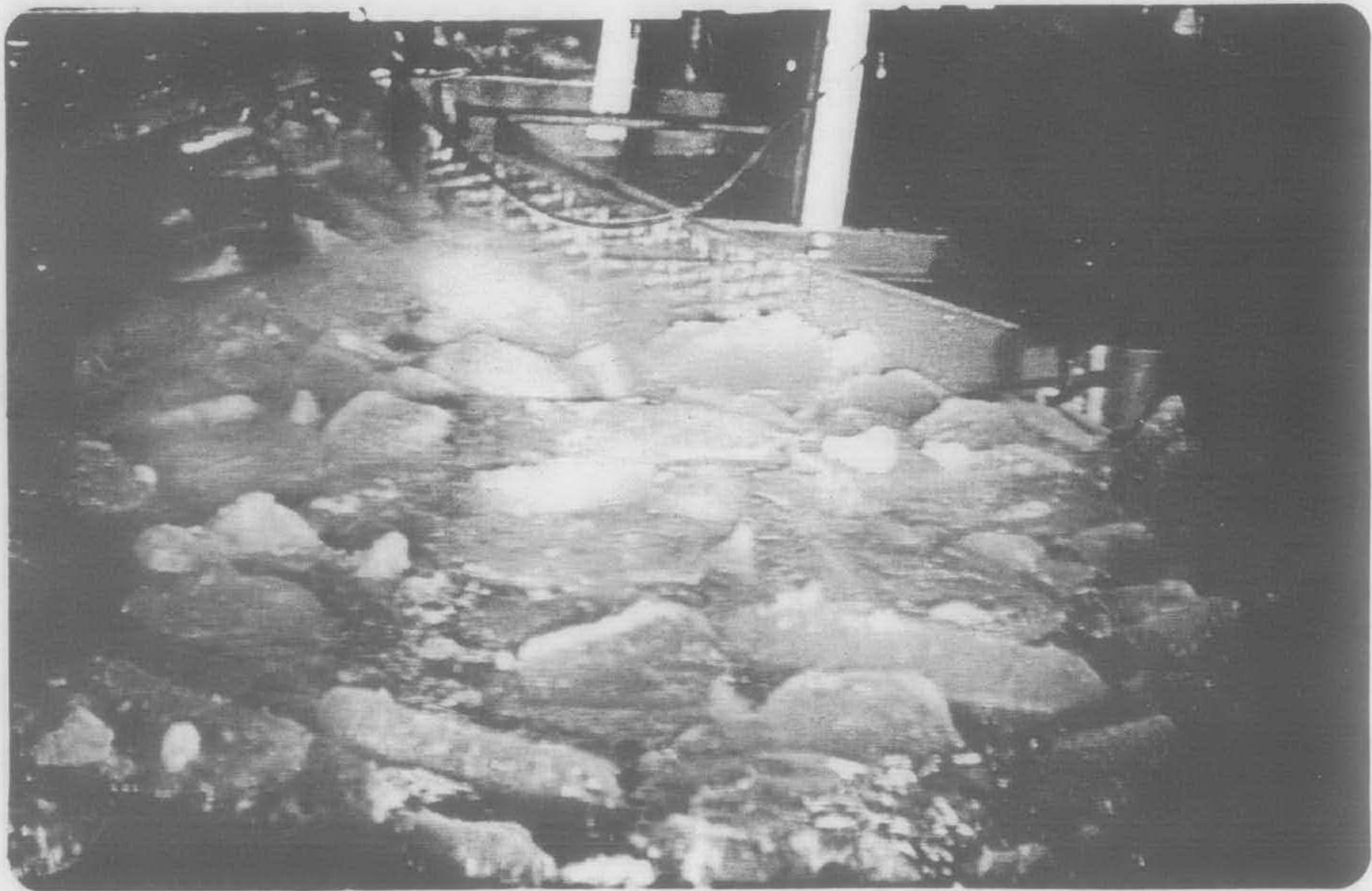
Figure 9. Test #6 in progress with a 5 mm oil slick, at 70% ice concentration.
