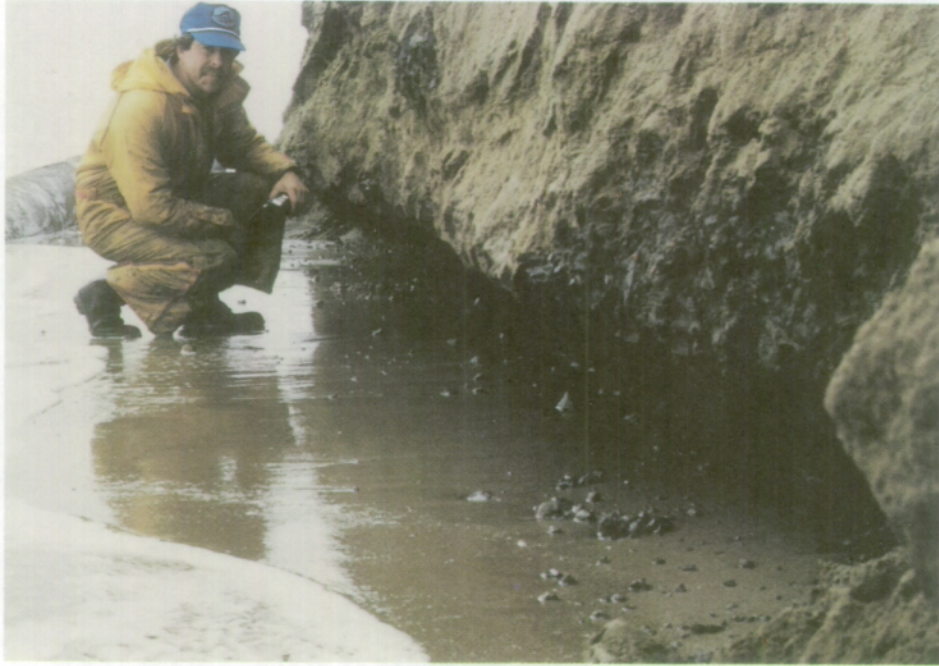
Figure 3.6 Undercutting of cliff base at waterline by thermo-erosion. The soil is frozen above the undercut. The undercut extends 1 to 1.5 m into the cliff base. (August 13, 1986).
