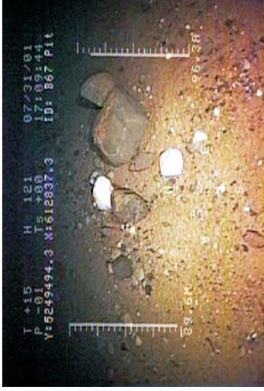
Figure D14: Large boulders on the lower inner berm with no biological growth.
